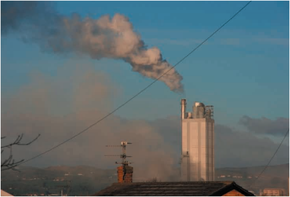
The Padeswood kiln was flushed on 27 March 2007. This is reportedly a frequent occurrence, despite Castle Cement's assurances that the problems have been addressed. Picture from www.cank.org.uk .
